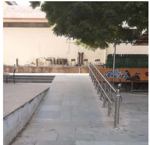
Ramp connecting the Canteen and new Academic Science Block
