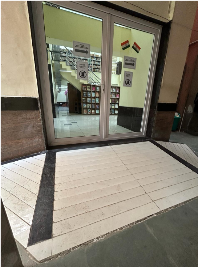
Front Entrance/Exit to the Library
